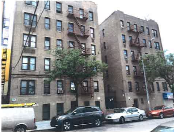
Figure 15: View looking South on West 169 th Street
