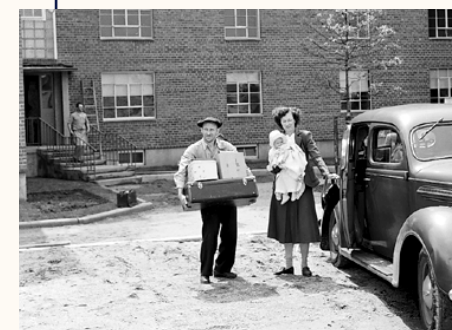
NYCHA Woodside Houses is constructed, featuring 20 6-story buildings over 22.3 acres.
