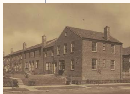
Sunnyside is developed as a low to moderate-density neighborhood of single-family homes and low-rise apartment buildings.
