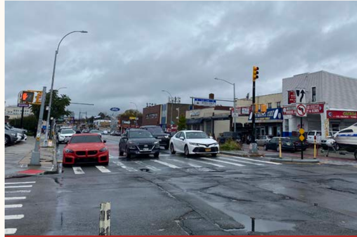
4. Improve the pedestrian experience by adding more crosswalks, shading, upgrading and beautifying pedestrian bridges and crossings, and repairing uneven sidewalks and sinkholes
