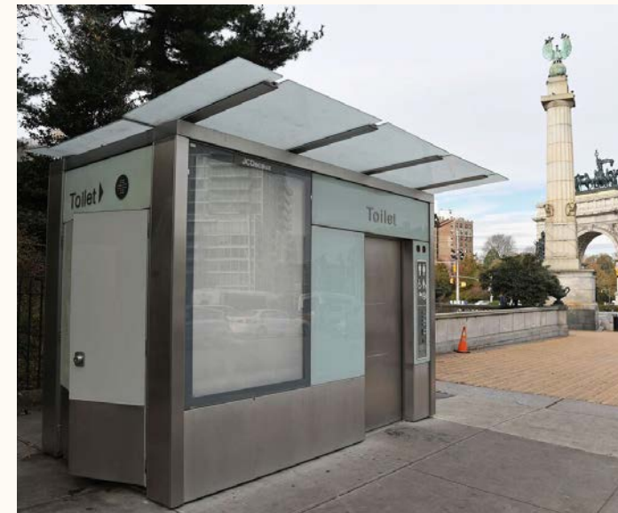
6. Create more accessible, clean public restrooms
