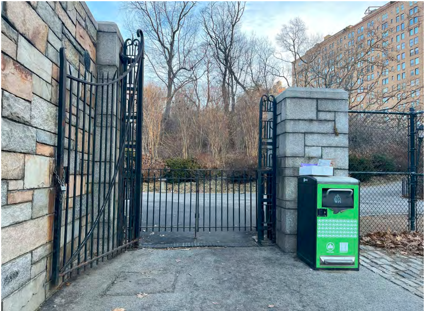
2 - Steel double entry gate (east side)
