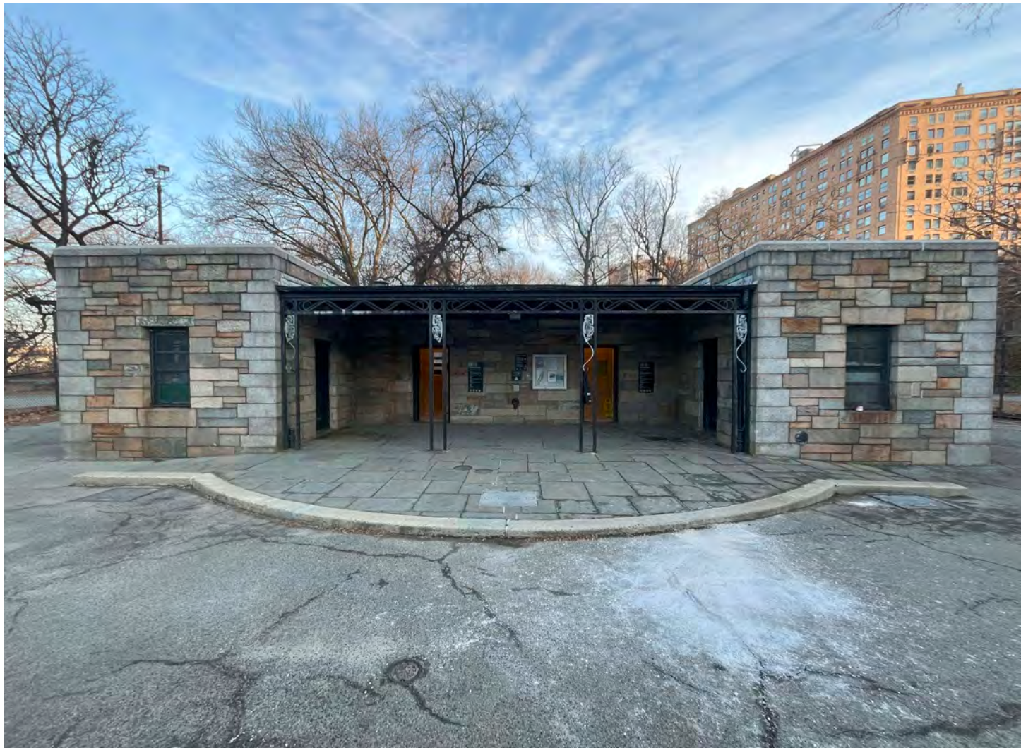
1 - South facade of public restroom building
