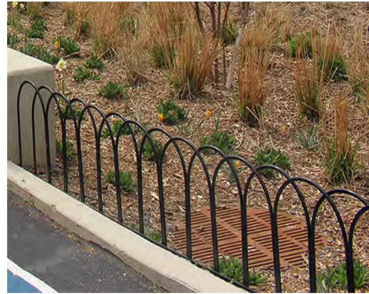
Wicket Steel Fence
