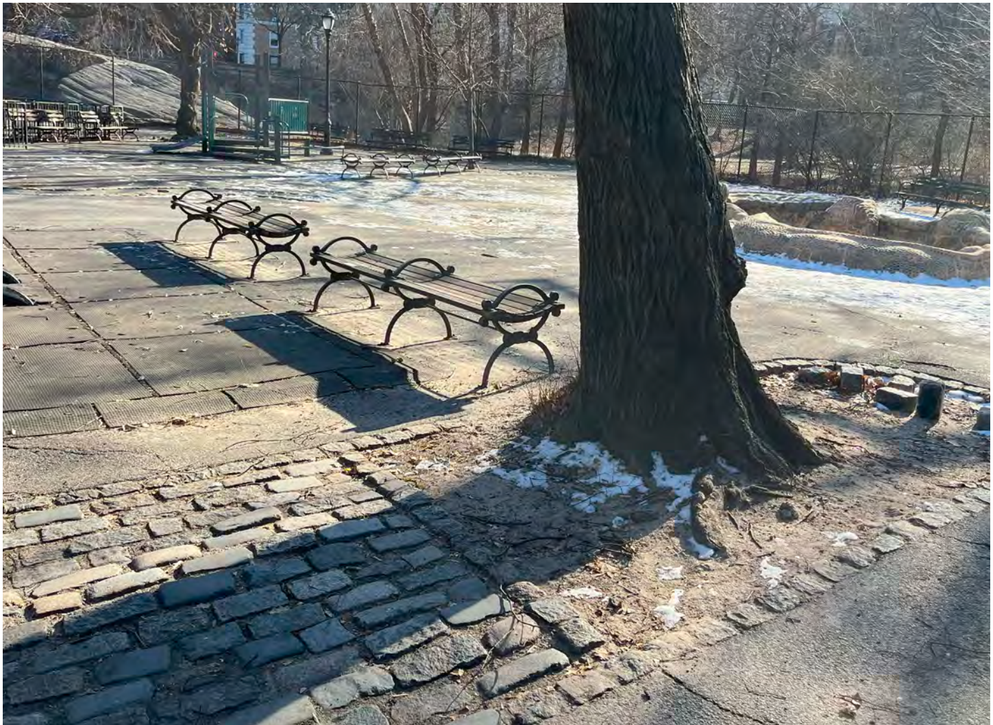
12 - Mature trees are in undersized tree pits bordered with granite block
