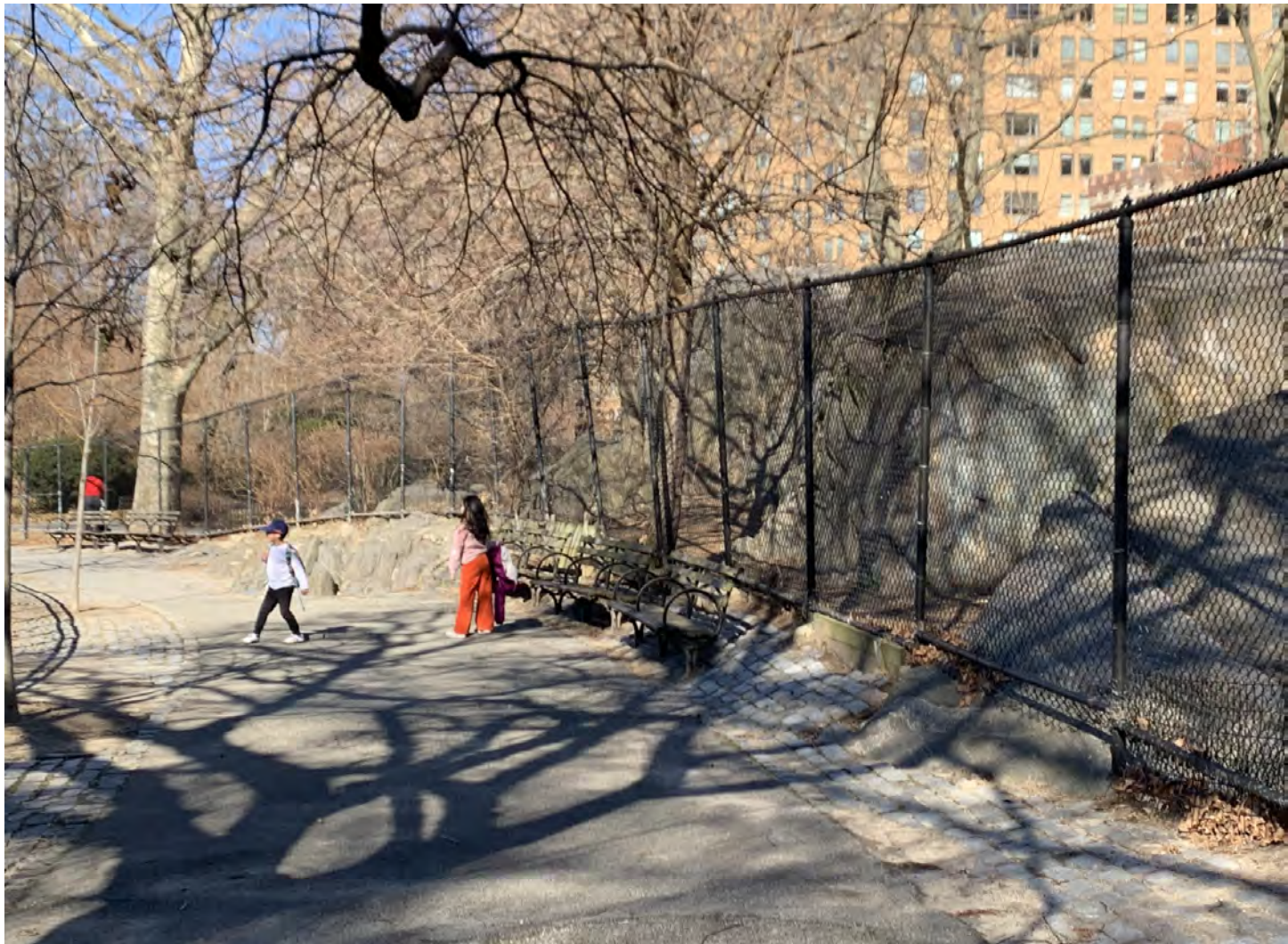
5 - Condition at northeastern perimeter
